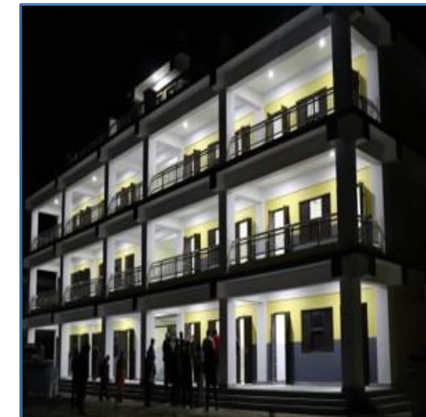
Reconstructed School Building Post Earthquake
